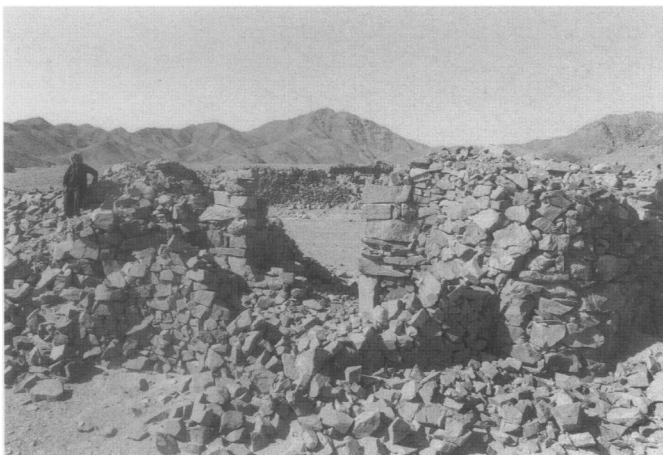
3. The gate in the southern wall of the hydreuma in Wadi Semna with flanking towers, looking northwest.
